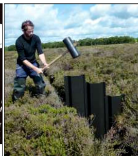
Actions include drain blocking to restore breeding habitat
